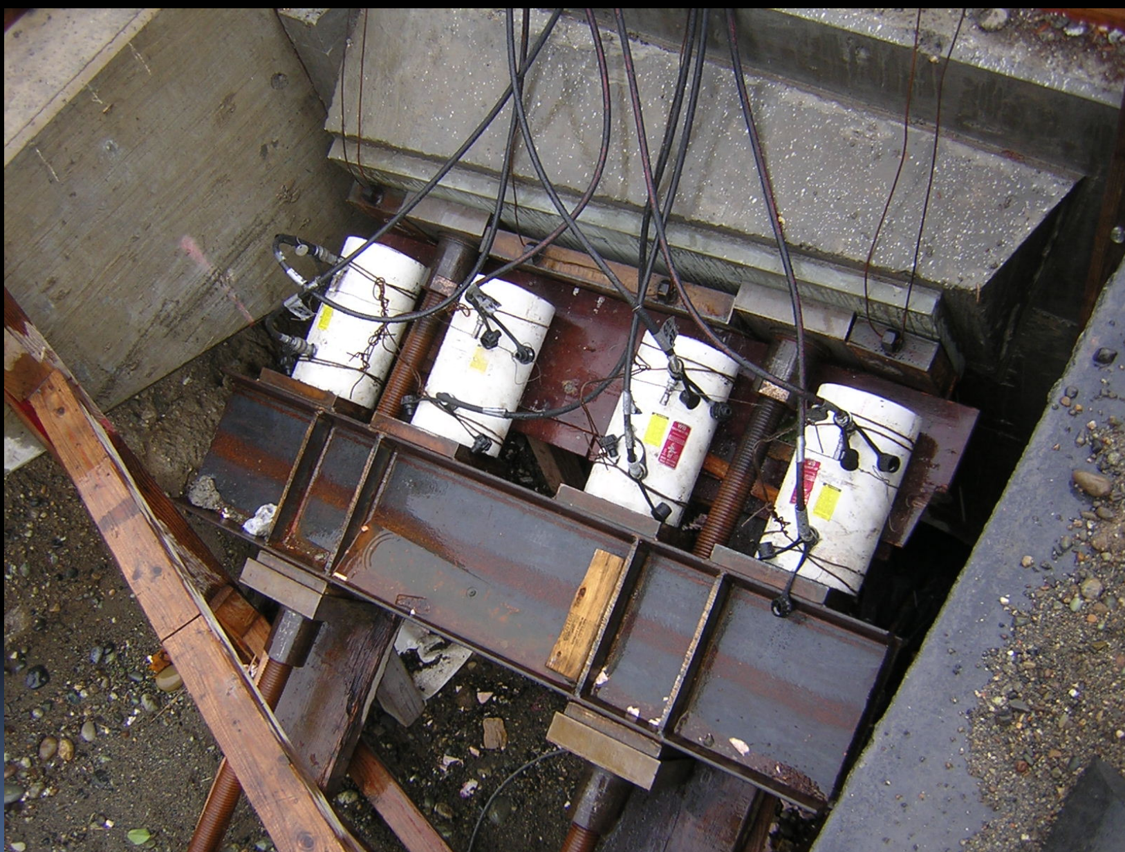
Backstay Jacking Station
